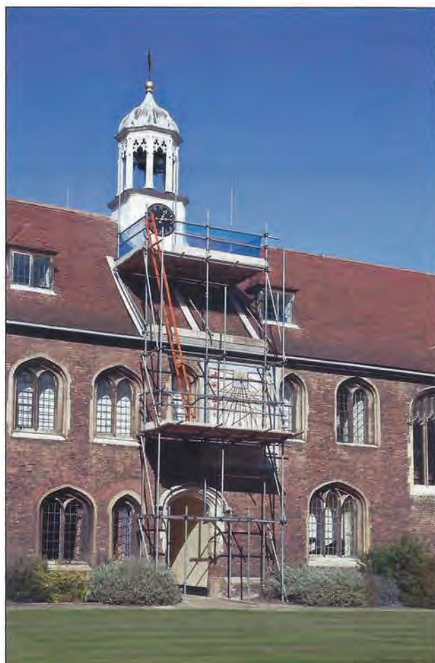
Scaffolding to repair the Clock Tower.
