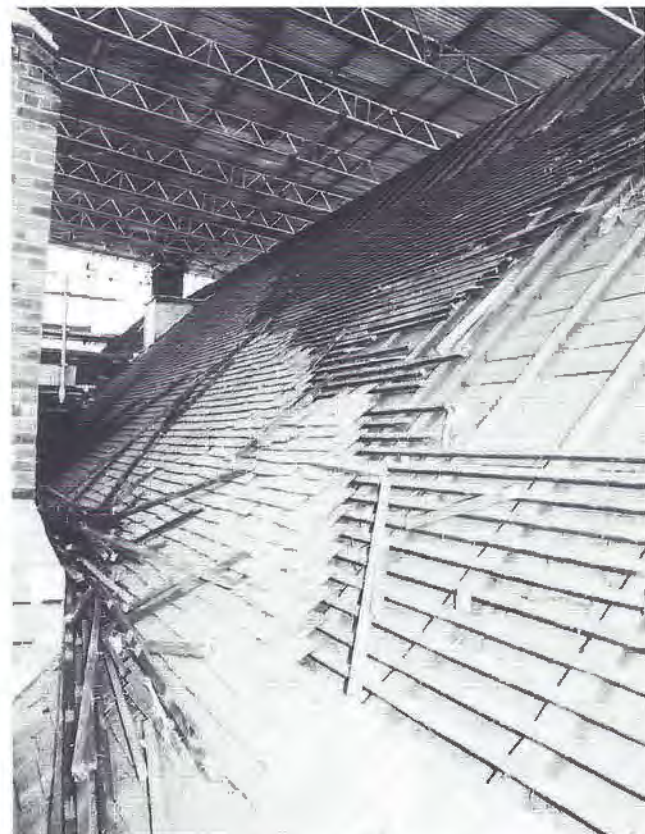
Removing the old slats and tiles, Old Hall.
