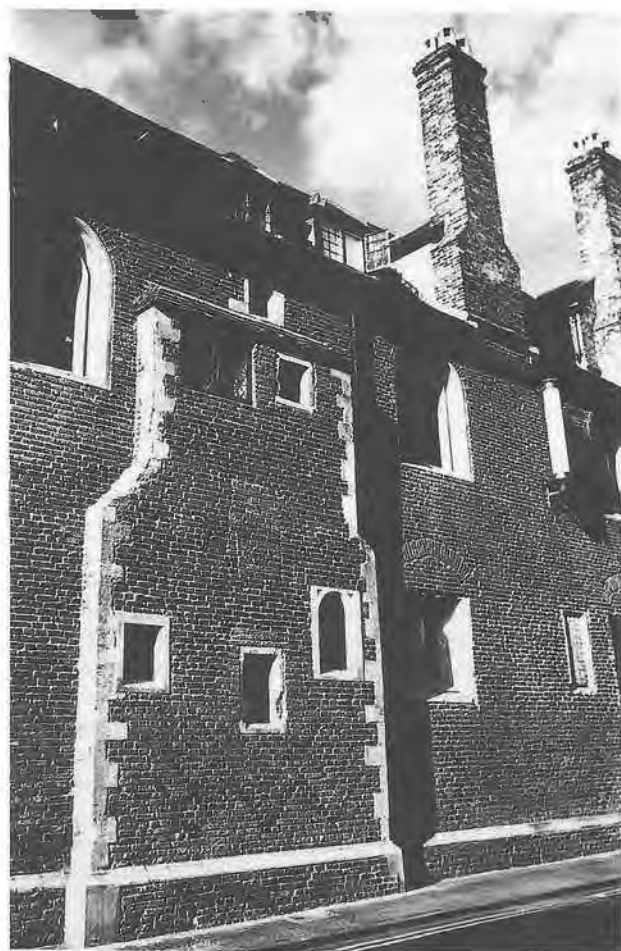
The recently restored Silver Street elevation of Old Court. Photo: Jonathan Holmes.
